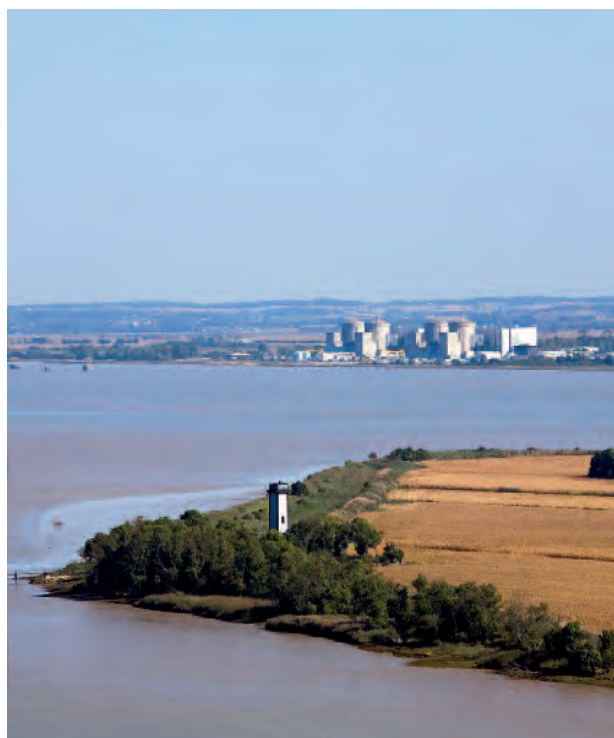
Aerial view of Le Blayais NPP, on the right bank of the Gironde estuary
