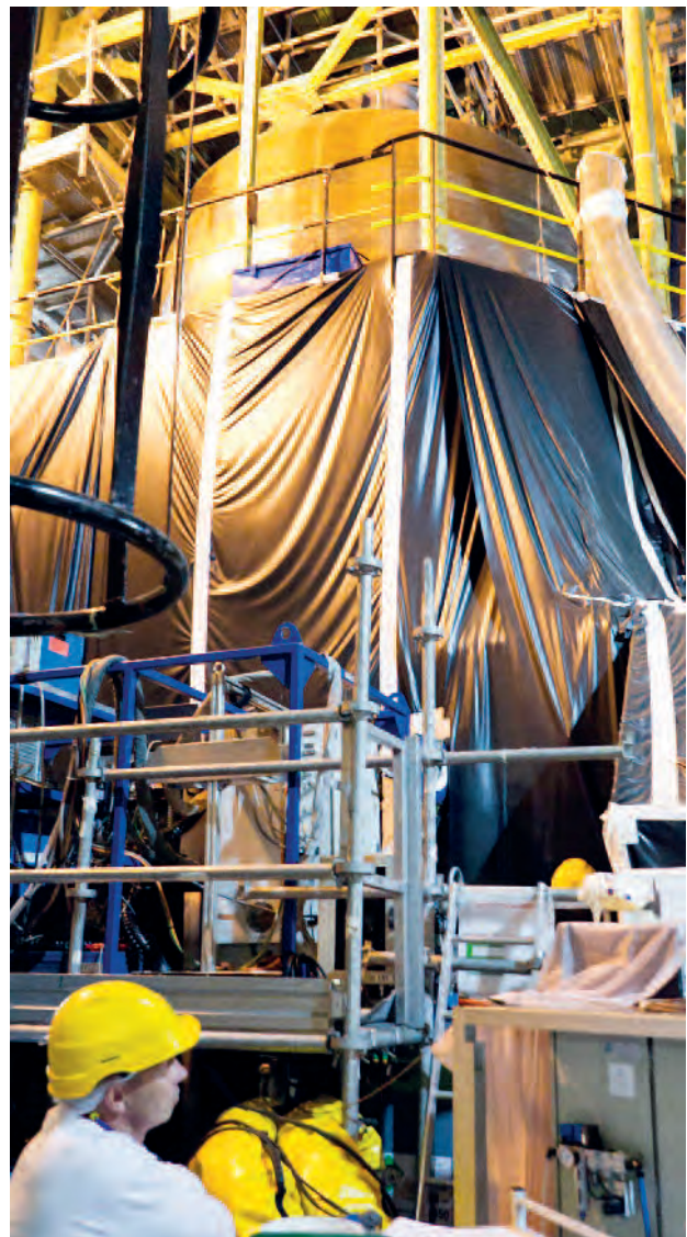
Monitoring of the steam generator replacement work on the occasion of the 3rd ten-yearly inspection of the Fessenheim NPP – September 2011
