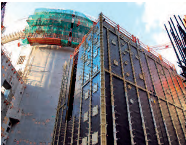
EPR fuel building spent fuel pool formwork panels – November 2010
