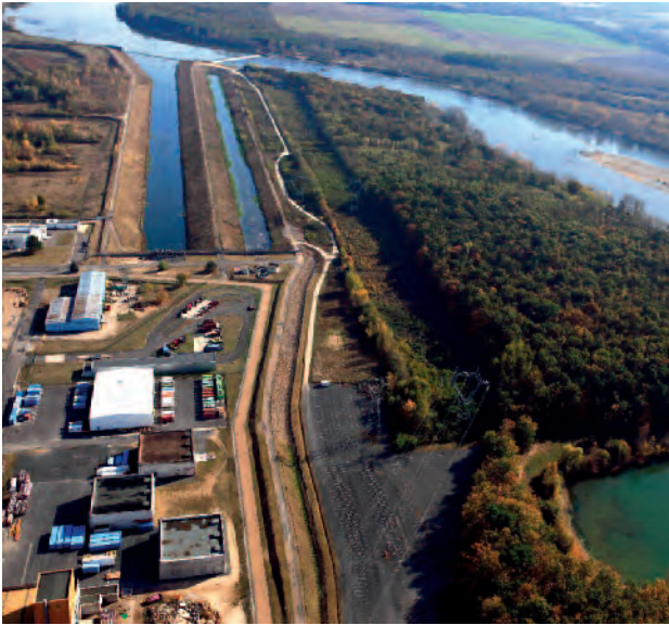
Water intake and discharge structures on the Loire river for the Dampierre en Burly NPP
