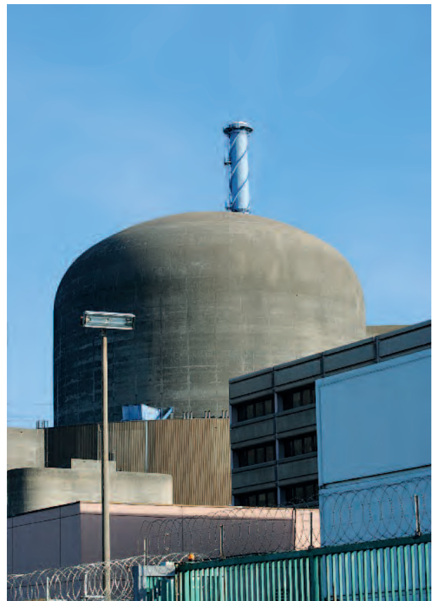
View of the concrete shell of the Flamanville NPP reactor building
