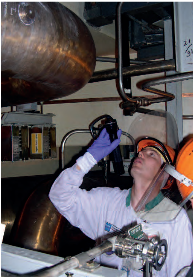
ASN inspection of a steam generator weld during hydrotesting of the primary system of the Cattenom NPP
