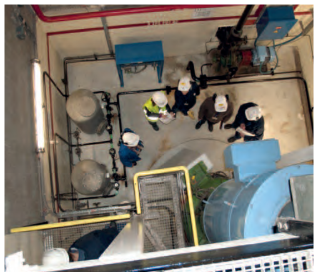
ASN inspection of the Cruas NPP pumping station
