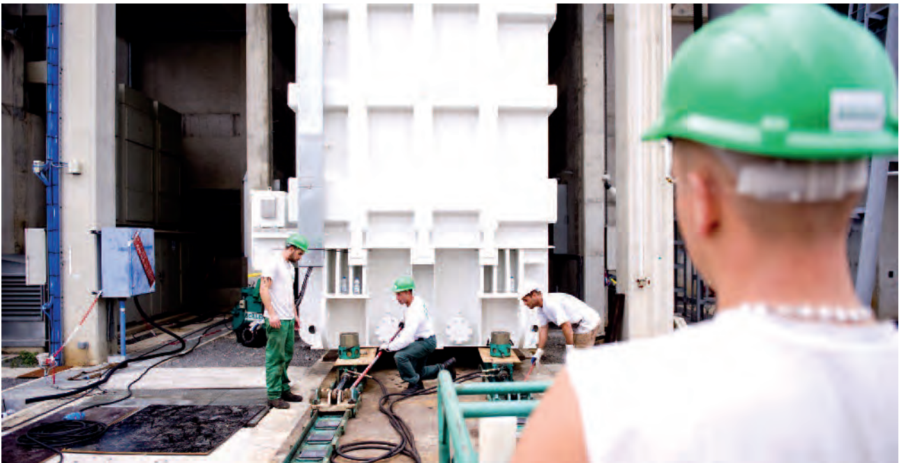
Contractors working on replacing the N4 transformer in the Civaux NPP – July 2009
