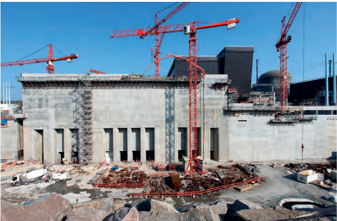
Start of the roofing work ending the civil engineering activities for the pumping station – April 2011
