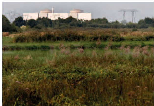
View of Le Blayais NPP
