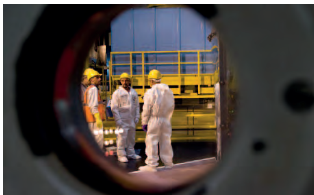
Maintenance in the reactor building on the Flamanville site during the reactor 2 outage
