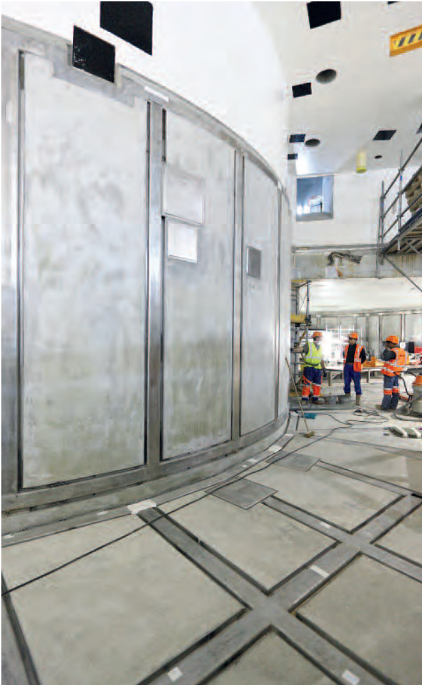
IRWST pool for the SIS system before sheeting
