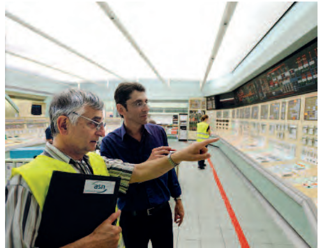
ASN inspection of the control room during the ten-yearly inspection of the Tricastin NPP – May 2009
