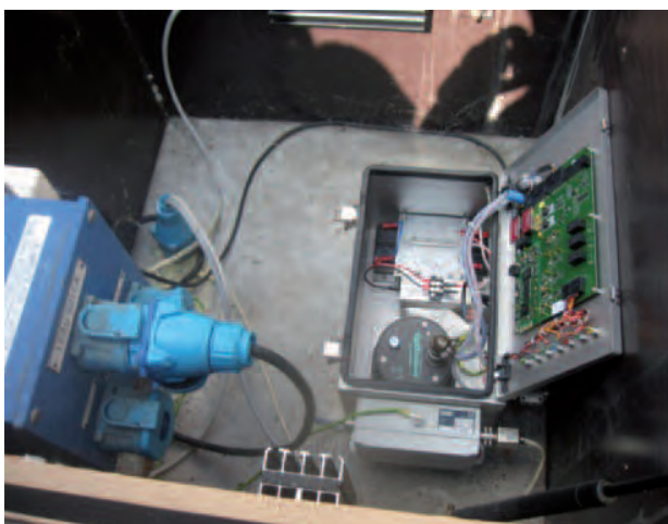
View of a seismic monitoring device (accelerometer) installed in an NPP
