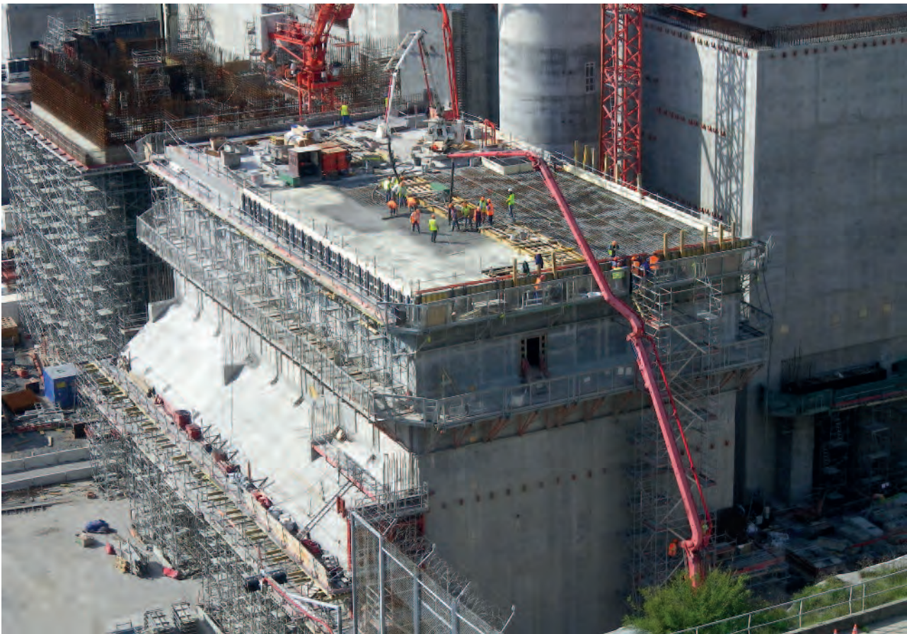
View of the south diesel building – August 2011
