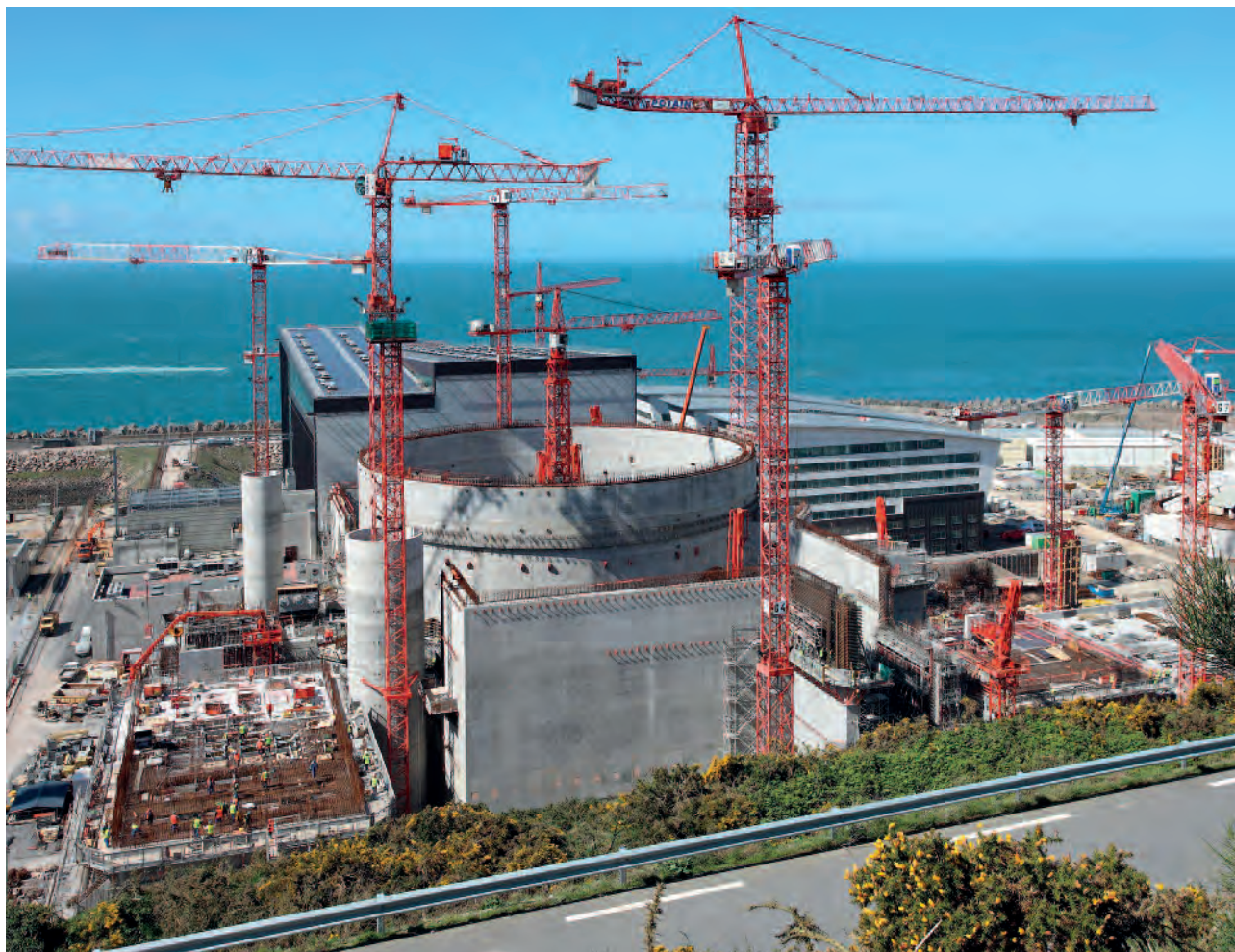
General view of the Flamanville 3 EPR construction site – August 2011
