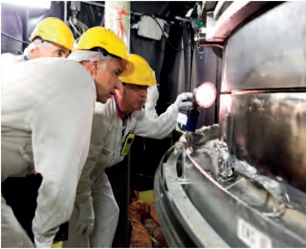
Inspection of an SG weld during the 3rd ten-yearly inspection on the Fessenheim NPP – September 2011
