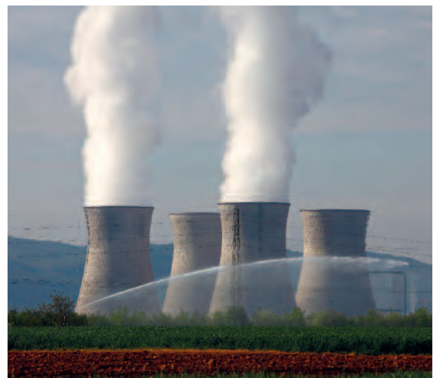
General view of the Bugey NPP
